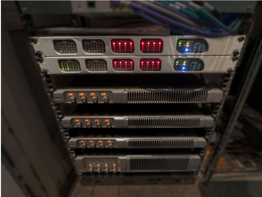
VMX88s doing their work in situ.
